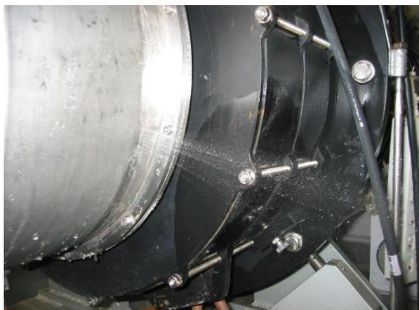
**Water leakage at klystron oil tank**
