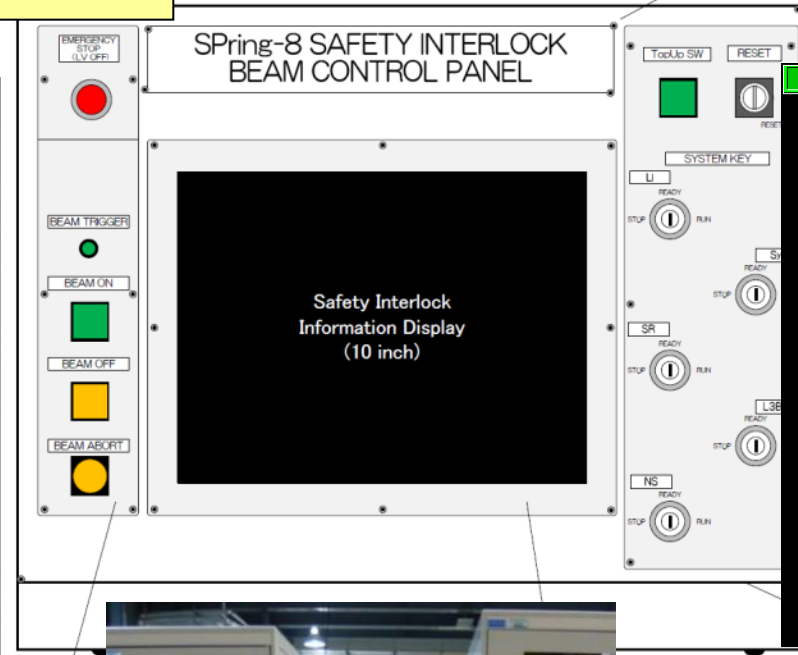
New Control Panel
