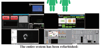
The entire system has been refurbished: Control system, Interlock, display, irradiation history, video stream of irradiation beam position.
